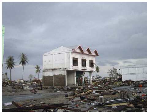
Tsunami inundation height can be seen on a house in Banda Aceh
